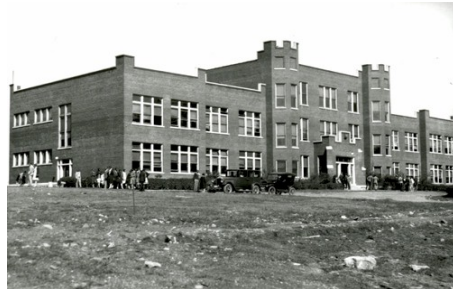
First Library in Main Building
